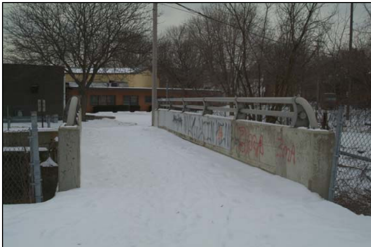
Existing Pedestrian Bridge Over Indian Mill Creek
